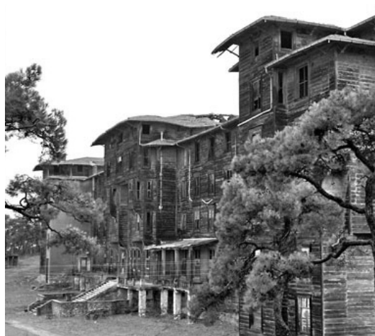
Former Orthodox Orphanage in Turkey
